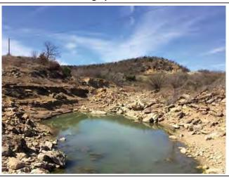
Facing upstream near middle of SAR. Note the high erosion and incision of the spillway channel below Lake Palo Pinto.
